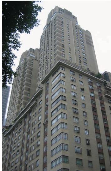
The Century Apartments by Irwin Chanin. Note the unique use of curtain wall windows and recessed openings. Photo credit: Anthony Robins.
