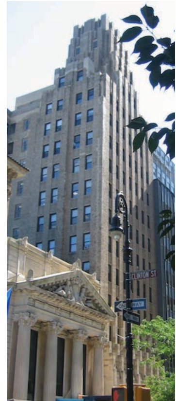
Brooklyn's National Title Guaranty Building emulates the vertical window placement and setbacks of its Manhattan predecessors. Its distinctive tile detail is not visible in this image. Photo credit: Anthony Robins.
