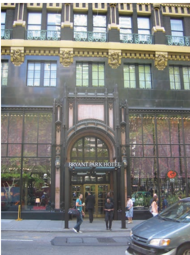
Raymond Hood’s American Radiator Building (now the Bryant Park Hotel), was the first New York skyscraper to use black and gold. Photo credit: Anthony Robins.
